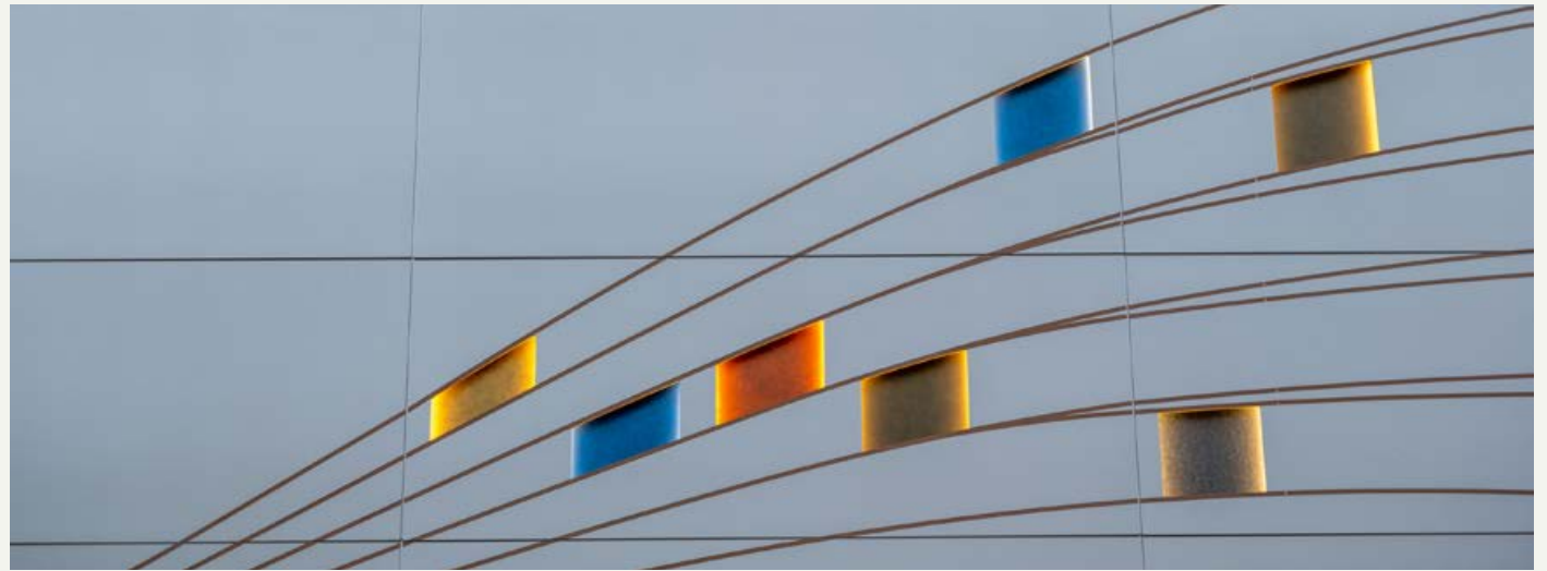
Rockpanel Headquarters, Roermond, The Netherlands
